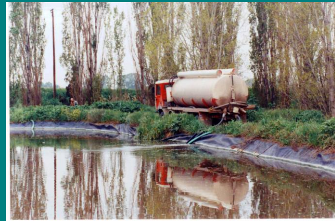
Septage disposal in a stabilization pond
